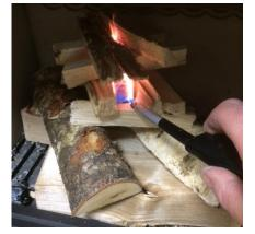
Light the firelighter(s), leaving the air control fully open and close the door. It should not be necessary to leave the door open but DO NOT leave the stove unattended if you find it necessary to leave the door ajar.
