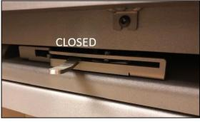
C) Sliding the operating rod across into the AUTO slot position where the rod will be depressed by the door as it closes causes the baffle flap to open when the door is open and closes it when the door is closed.
