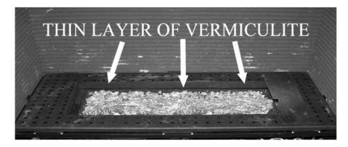
Place a thin layer of Vermiculite on top of the Stainless Steel burner as shown, avoid blocking the Pilot Assembly. (LPG ONLY)
