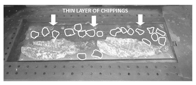
• Place a thin layer of black chippings on top of the Stainless Steel burner as shown, avoid blocking the Pilot Assembly. (NG ONLY)
