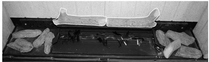
Place two log shapes upon the shelf above the inlet baffle as shown. Place a further two log shapes along the front edge of the burner cover.
