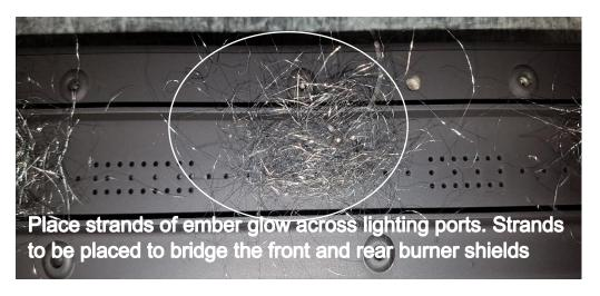
Within this packed appliance is one packet of Ember glow. Only half of the packet should be used per install, the spare half of the pack is provided for the first annual service. Failure to place the correct amount of flakes and in the correct burner area can result in producing a poor flame picture and sooty deposits.
