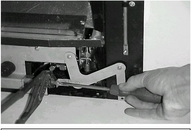
Check for gas soundness. Reconnect the bell crank mechanism as above ensuring that the gas control spindle is gripped only over the protective copper sleeve and no other part of the spindle as, ensure NO side strain is applied to the spindle.
