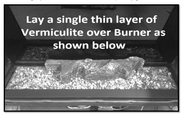
• Make sure not to block around the pilot area on the Burner and Front Infill cover, if flakes fall in, it may be worth lifting the Infill grill out carefully and removing, before carrying on with laying the shapes.
